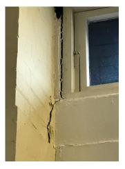
This picture of the cracking shows the top part of the supporting pier and the window frame that appears to be pulling away.
